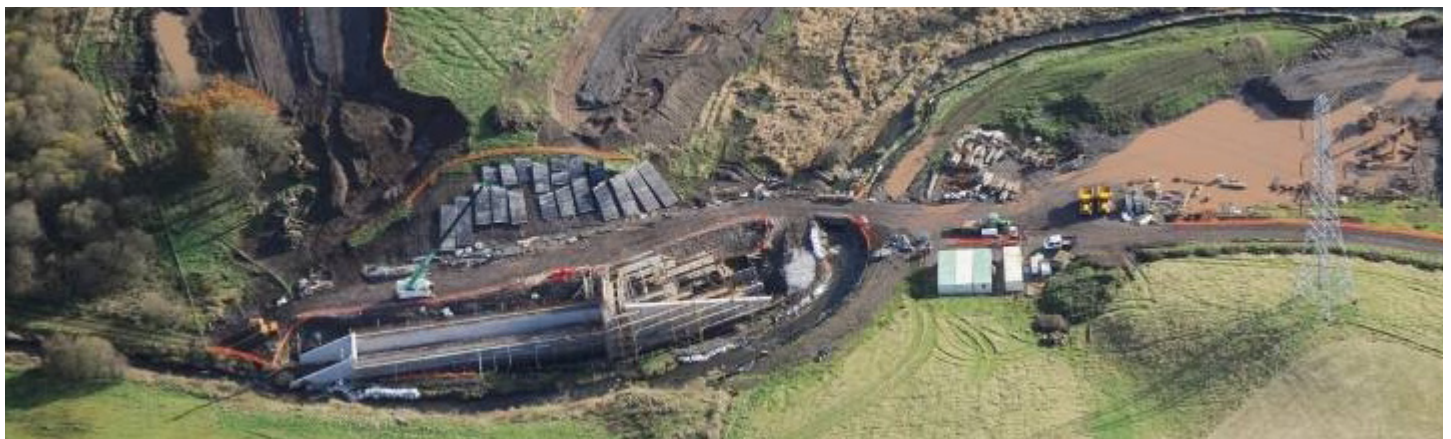
One of three new flood storage areas being built to control the surge of flood water upstream before it flows towards urban areas
