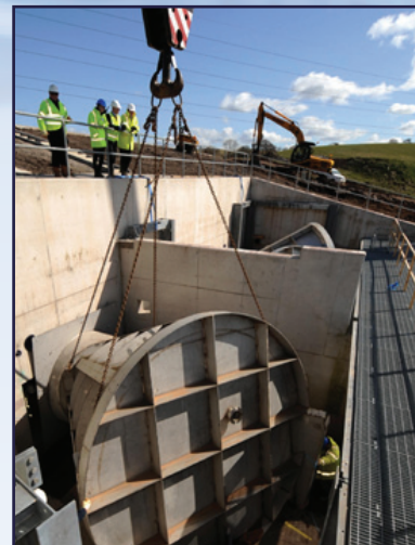
White Cart “hydro brakes” being installed
