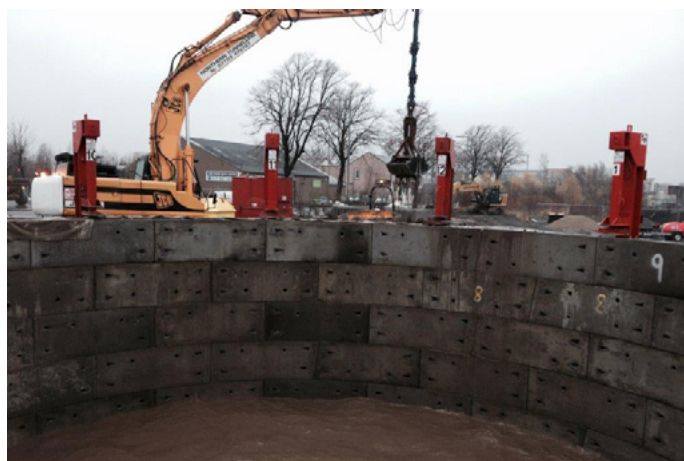
Caisson excavation jacking
