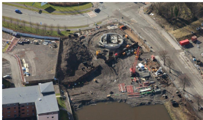
Aerial view of caisson construction
